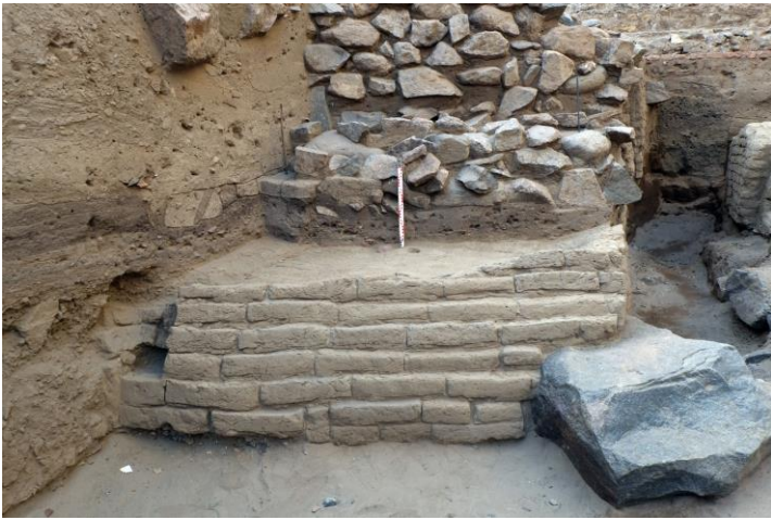
Fig. 9: Area 3: View of the northern face of the retaining wall of Stratum M.
